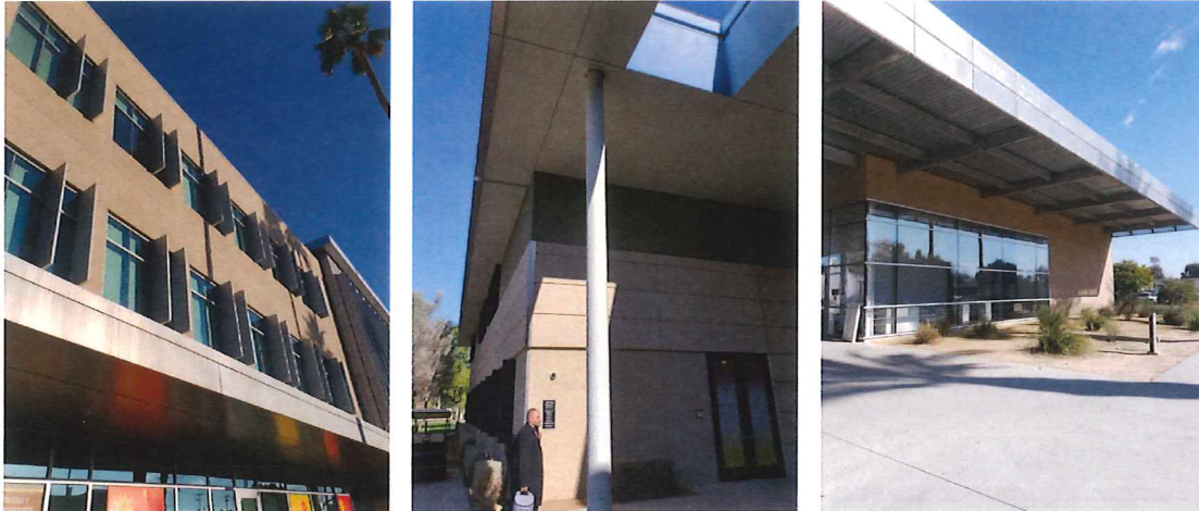
IMAGE 1.13 | SOLAR SHADING EQUIPMENT (INDIO & PALM DESERT CAMPUS)
