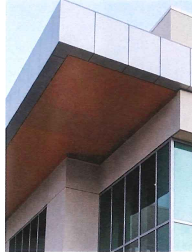
ALTERNATE 3 - PLASTER PANEL INFILL
