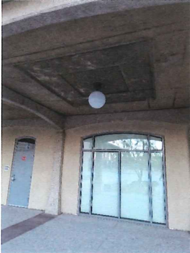
REPAIRED CONCRETE SOFFIT
