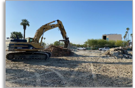
Site Demolition & Clearing
