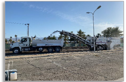
Site Demolition & Clearing
