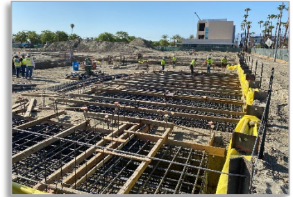
Rebar for Structural Footings
