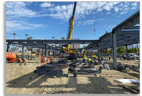
Steel Erection
