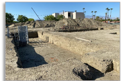
Underground Utilities & Footing Prep
