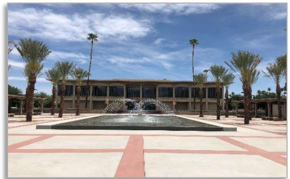
Central Campus Quad Renovation
