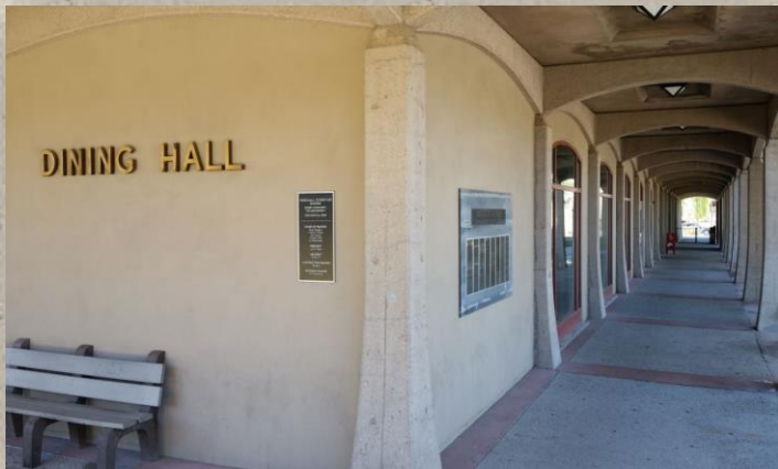
Dining Hall Renovation
